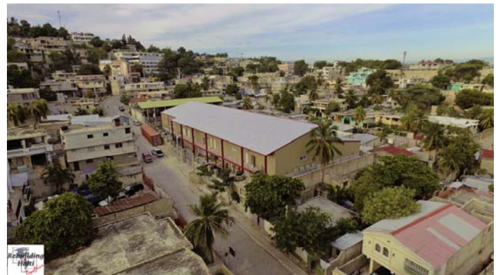
(Delmas 9, Aerial of completed project.)
